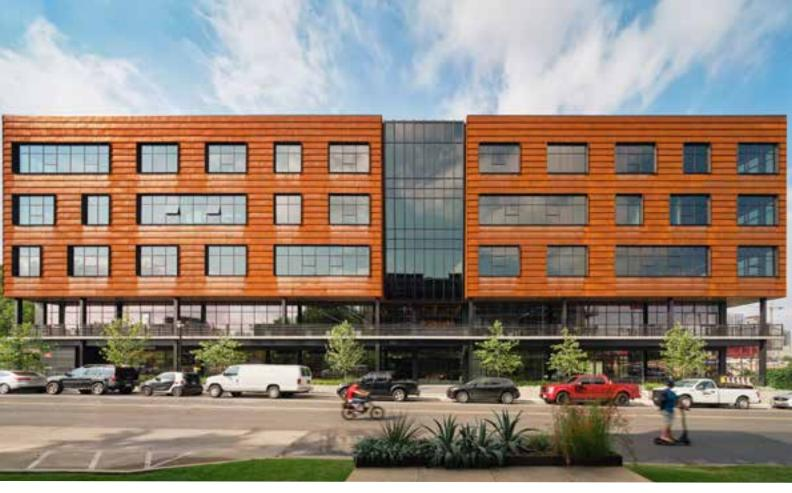
In the elevator cabs, the design team licensed woodcut relief prints from the estate of artist Bryan Nash Gill, which were installed as dramatic backlit panels on the rear walls. The building is clad in a distinctive tapered Corten panel, while a wraparound balcony at the second level gives added depth to the street-facing facade.
