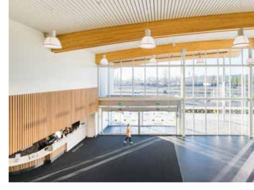
The 33 trusses were prefabricated in halves at the engineer's shop to allow for efficient erection on-site. The double-span roof panels, composed of exposed timber purlins and plywood that meet heavy timber requirements, were also prefabricated quickly in the shop, in widths to suit the curvature of the roof. Spruce glulam was used, allowing the lighter tone of wood to create a beautiful contrast with the black-painted steel webs.
