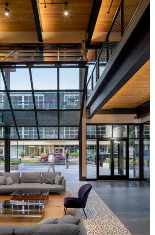
The building is the first in Texas to use CLT as part of a composite structural system. At the double-height entry lobby, a 25-ft. bi-fold door allows the space to be opened dramatically to the street during special events while serving as a showcase window for the CLT, which is visible at the ceiling and in a full-height "feature wall" assembled from waste off-cuts.
