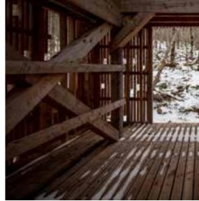
Refuge is made of rough-sawn spruce timber. To protect the spruce from the elements, a bitumen waterproofing was placed on the reverse board and batten wall, and on the roof envelope. The structure has a very taut skin with no overhangs and a skirt that is scribed to the ground; this is done to minimize the effects of extreme uplift from the prevailing *suêtes*. Openings in the hut are small, creating a dimly lit space.
