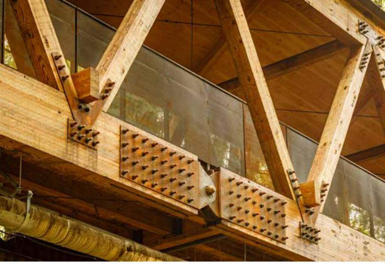
The parallel chord wood trusses needed to span the ravine were about 12 ft. tall and spaced to straddle the existing bridge deck and utilities when craned into place. This allowed for a critical installation sequence that transferred the support of the utilities from the existing bridge deck to the new structure, keeping the utilities active and at the same elevation. The
