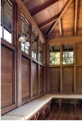
ulia Morgan Hall at University of California (UC), Berkeley, is an elegant redwood bungalow with natural-finish redwood interior and exposed structural wall and roof framing. The interior relies on the simple but beautiful exposed wood framing and wood detailing to create a warm and inviting space.
