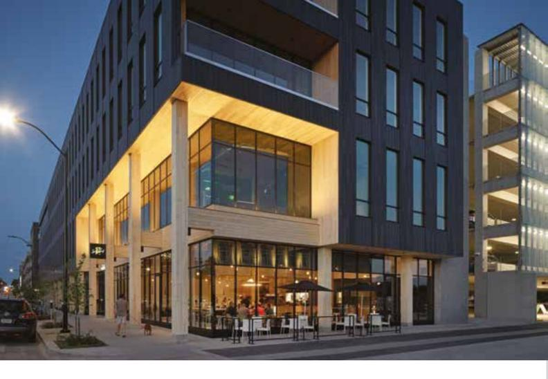
A four-story, mixed-use mass timber building with both retail and office space, its columns and beams are of glulam construction. The height and construction type (III-B) enable all levels to be of mass timber construction with a one-hour fire rating separating the first and second levels. Precast concrete panels compose the south portion of the building where the service core is located, creating a
