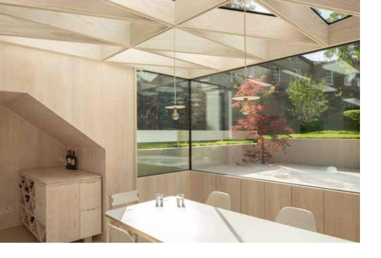
The design also benefits from the natural structural capacity and low thermal conductivity of wood. The design team simplified a conventional layered arrangement of a building envelope (structure, insulation, cladding) into one solid wood piece to form the entire structure and enclosure, with glazing units in four-seasons glass. Although each section needed to be wide and deep, they contribute to establish the character of the space
