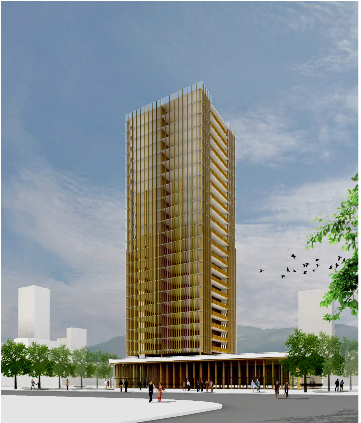
Option 2 illustrated with a glulam curtain wall and podium base
