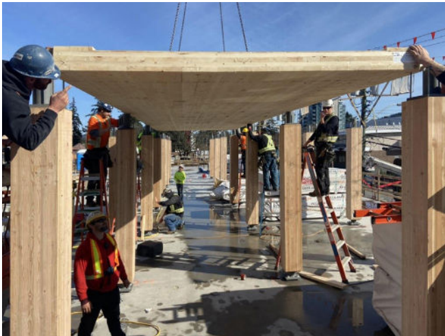
Figure 1. Tallwood 1 – installation of first CLT panel, March 2021
