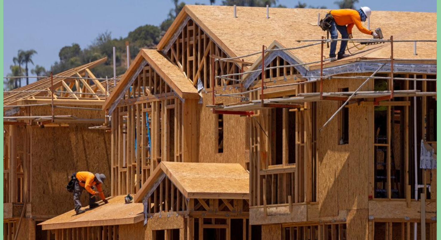
Construction workers in the process of building a traditional wood framed house
