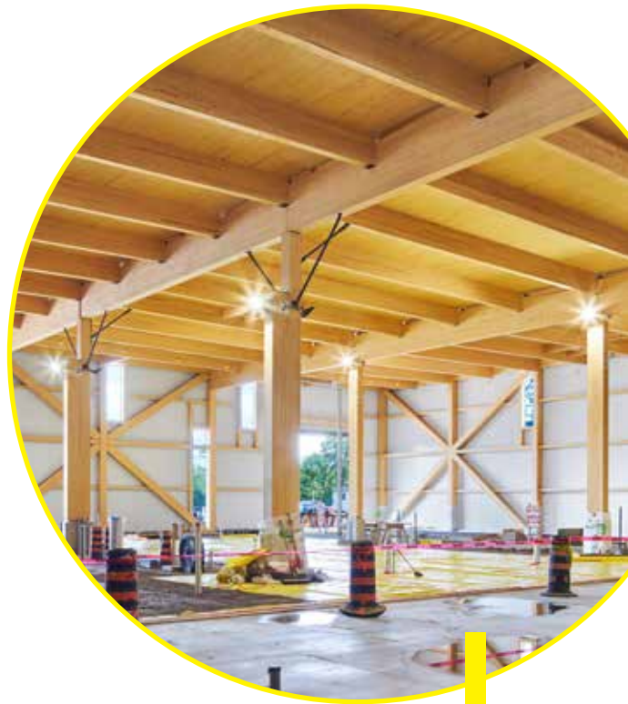
Figure 2. The Support Facility
