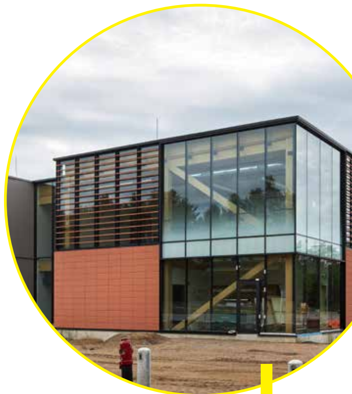
Figure 3. Minwamon Building (formerly called "Logistics Warehouse")
