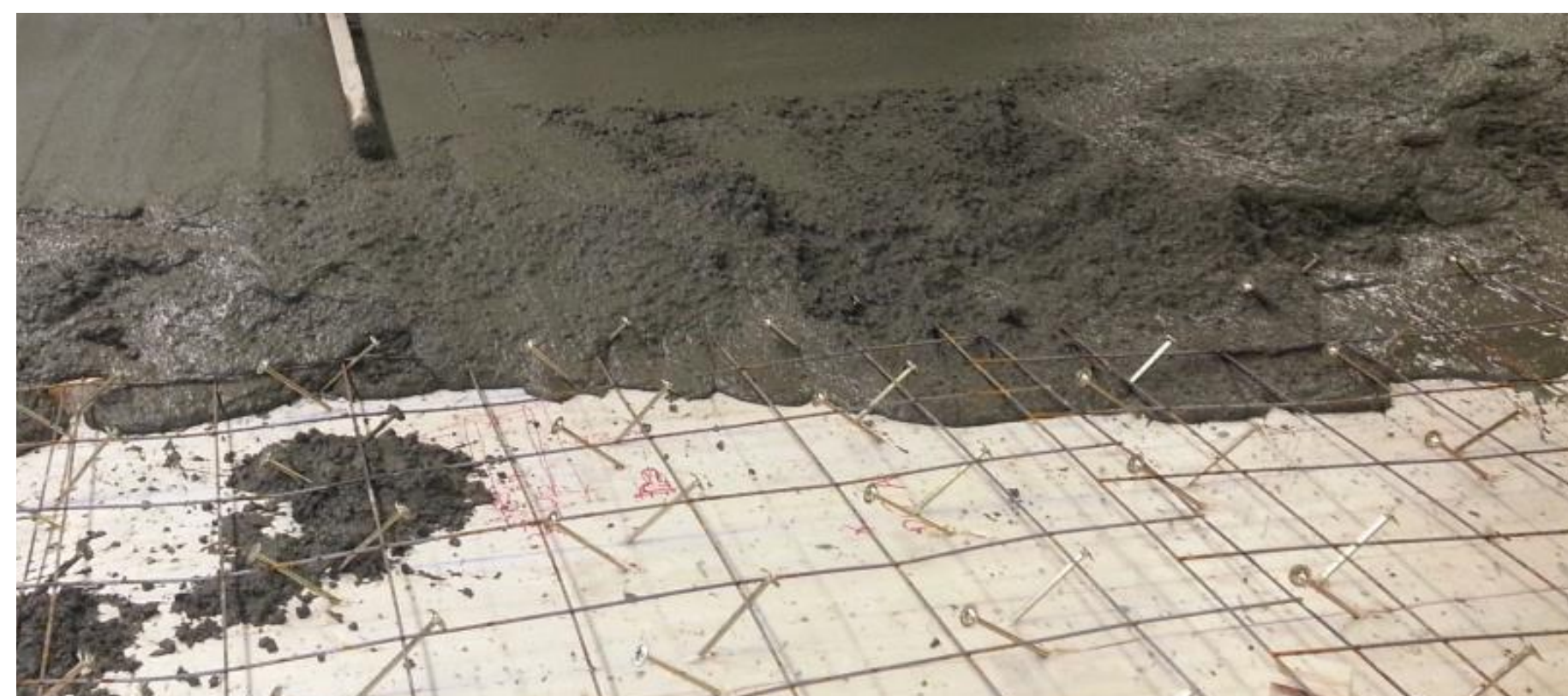
Self-tapping screws installed at 45°
