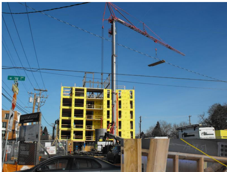
6-storey CLT building with a steel LLRS, Portland, Oregon
