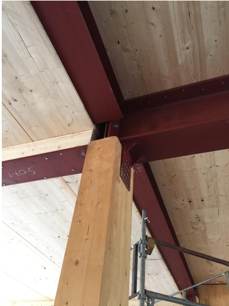
Steel floor beam with timber columns and CLT floor deck
