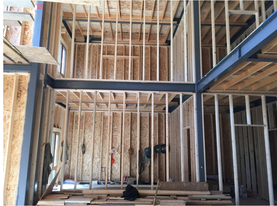
Steel frame building with light wood floor and wall panels
