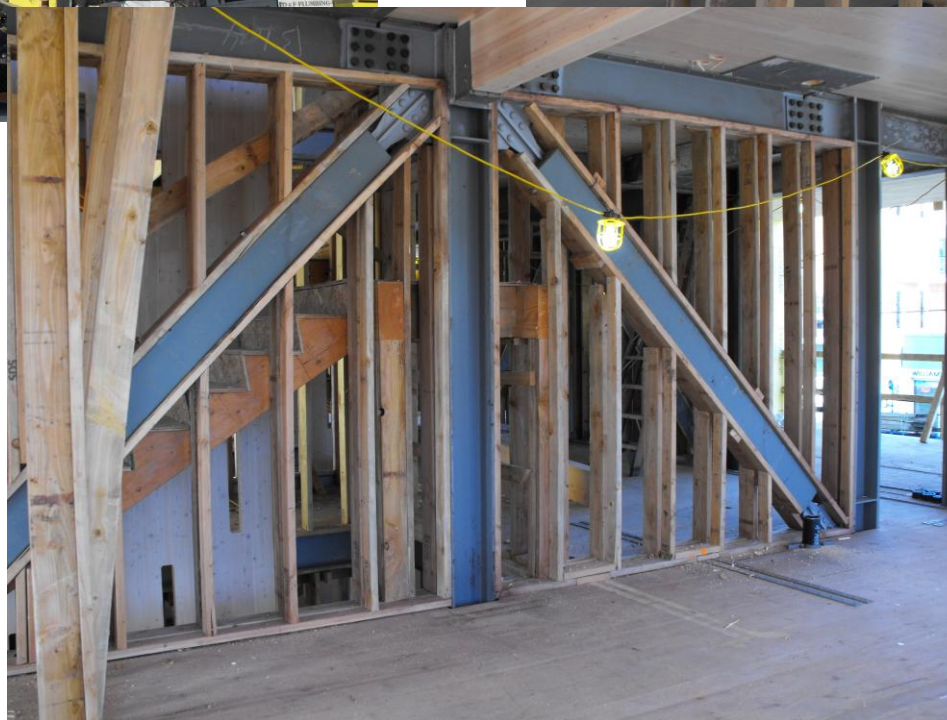
6-storey CLT building with a steel LLRS, Portland, Oregon
