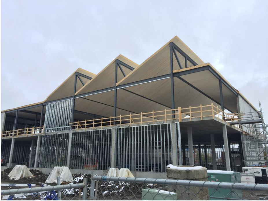
Steel frame structure with CLT roof panels (MEC Building, Edmonton)
