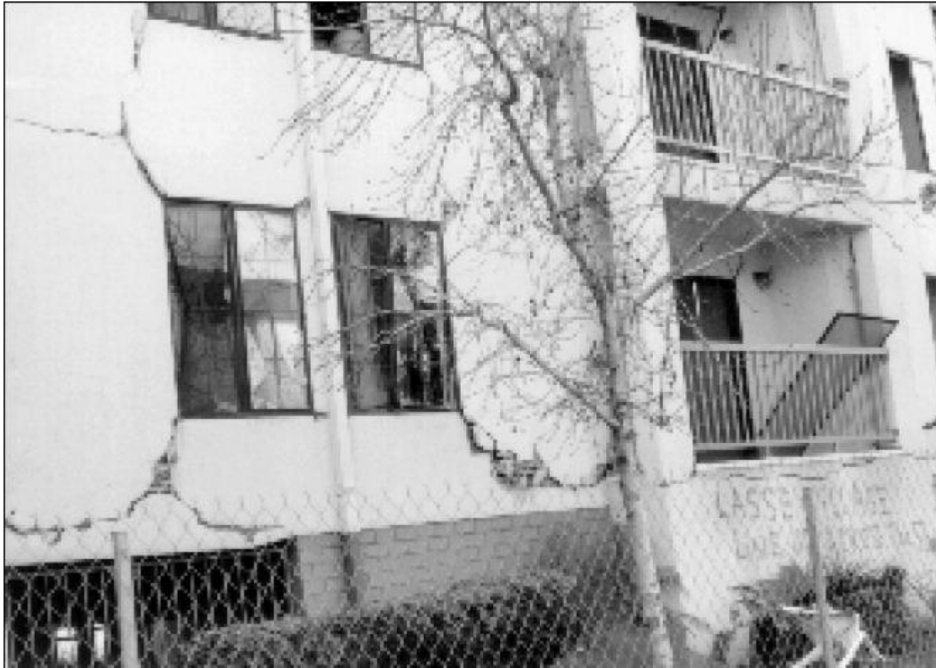
Stucco failure
