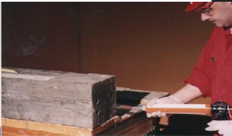
3. Injection of resin (epoxy glue)
