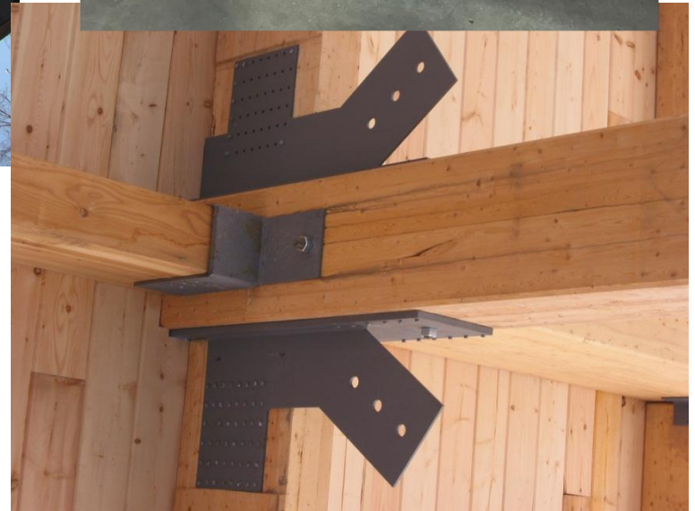
Timber rivets in a steel-wood connection
