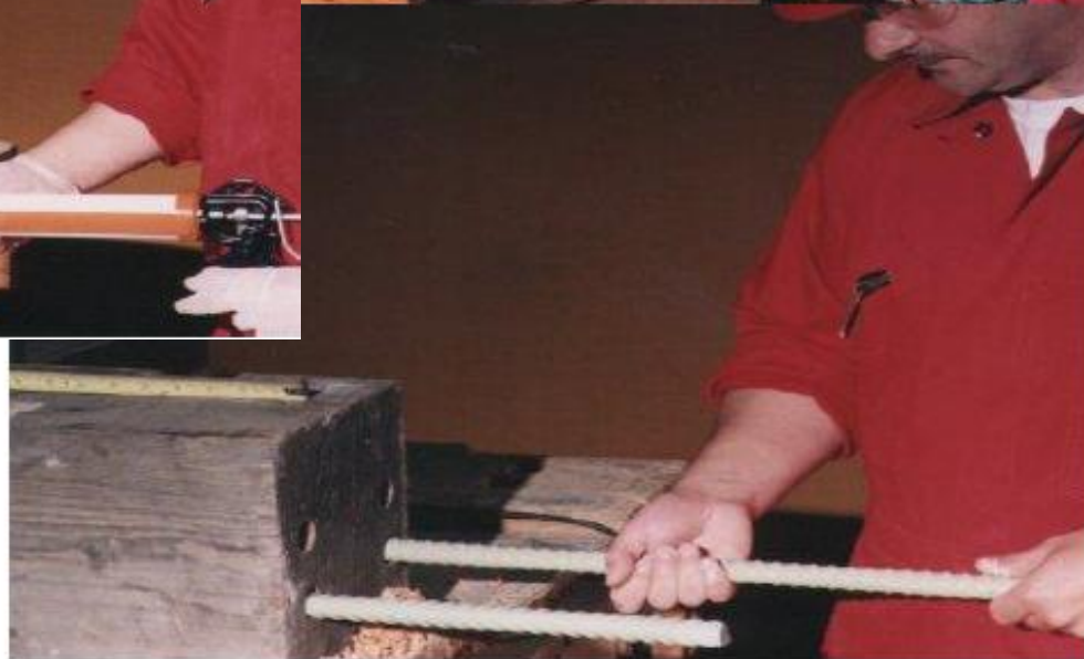
2. Threaded steel rod installation
