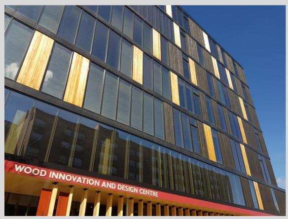
Facades exposed to rain (here the WIDC) can be protected from moisture by various coating, such as paint, oil finish or Nano coatings. A historical method experiencing a renaissance over the last 20 years in Europe and North America is charring.
