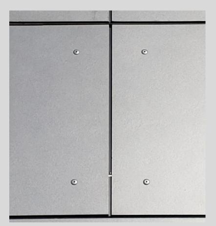
Cement Fiber Board Façade of the Wood Innovation Research Laboratory (WIRL) in Prince George. The open cladding allows for high drying potential. Perforated metal sheeting keeps insects and rodents out.
