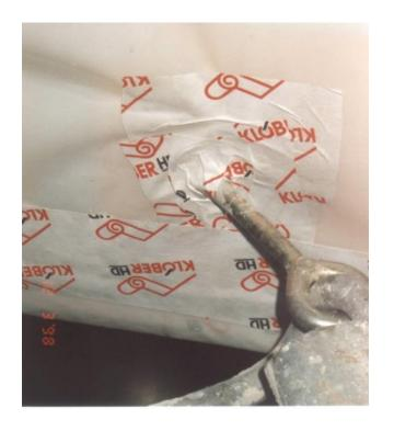
The material costs for appropriate Gaskets might be higher than for the tape but if possible, proper Gaskets should be used.
