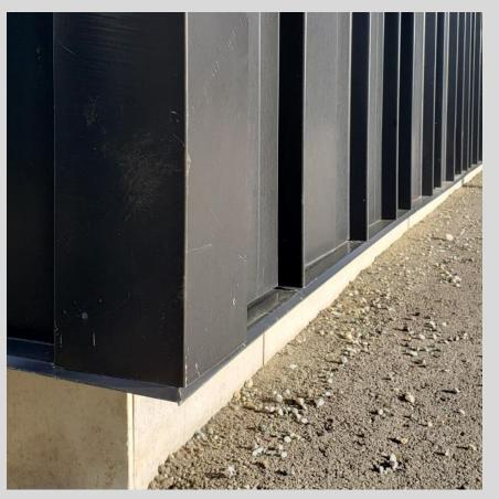
Metal Façade of the Wood Innovation Research Laboratory (WIRL) in Prince George. The very limited ventilation layer of only 19mm and extremely small openings does not allow for much ventilation. Not advisable in more humid climate zones and/or buildings with higher internal moisture loads.
