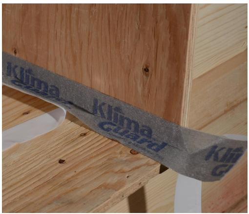
Corner tapes have two strip backing, so that one can be pulled of and glued down and then the second backing can be removed to finish the seal.
