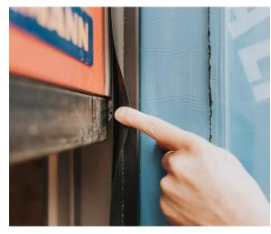
EPDM layer reduces friction of seal against door
