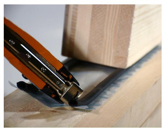
Tape with two hollow rubber hoses to seal gap between floor and walls, staples on wood to achieve airtightness.
