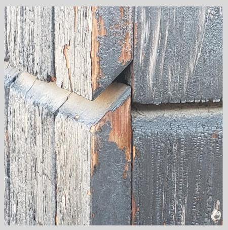
Base of the Wood Innovation Design Center (WIDC) in Prince George. The bottom 300 mm are sacrificial and could be replaced. The close-up also shows the shortcoming of the charring technique used in this particular case.
