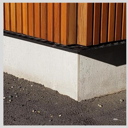
Base of the Wood Innovation Research Laboratory (WIRL) in Prince George. Mineral Boards cover the first 300 mm to protect the insulation behind and keep the wood façade out of the "splash zone".
