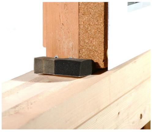
Compressed Foam tape self expands after installation (30-90min, depending on temperature), achieving airtightness with defined vapour diffusion resistance.
