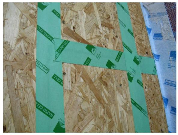
OSP has a relatively rough surface and need specific tapes with a relatively thick adhesive layer and flexible consistency to properly seal all micro gaps
