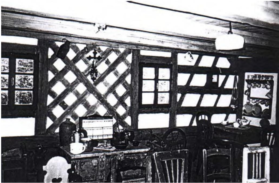
Half-timbered wall [1]
