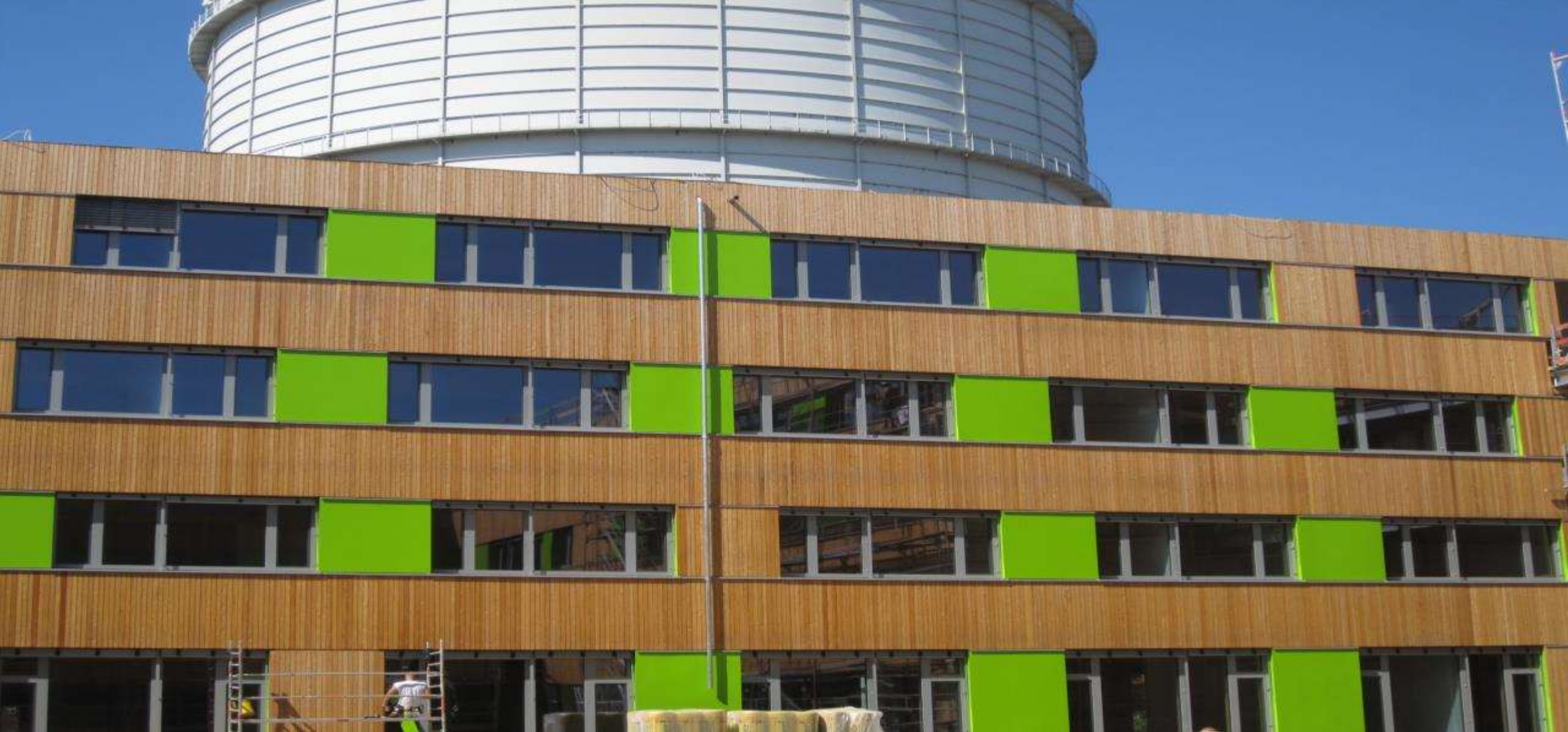
OFFICEBUILDING PUBLIC SERVICES LÜBECK/GERMANY
