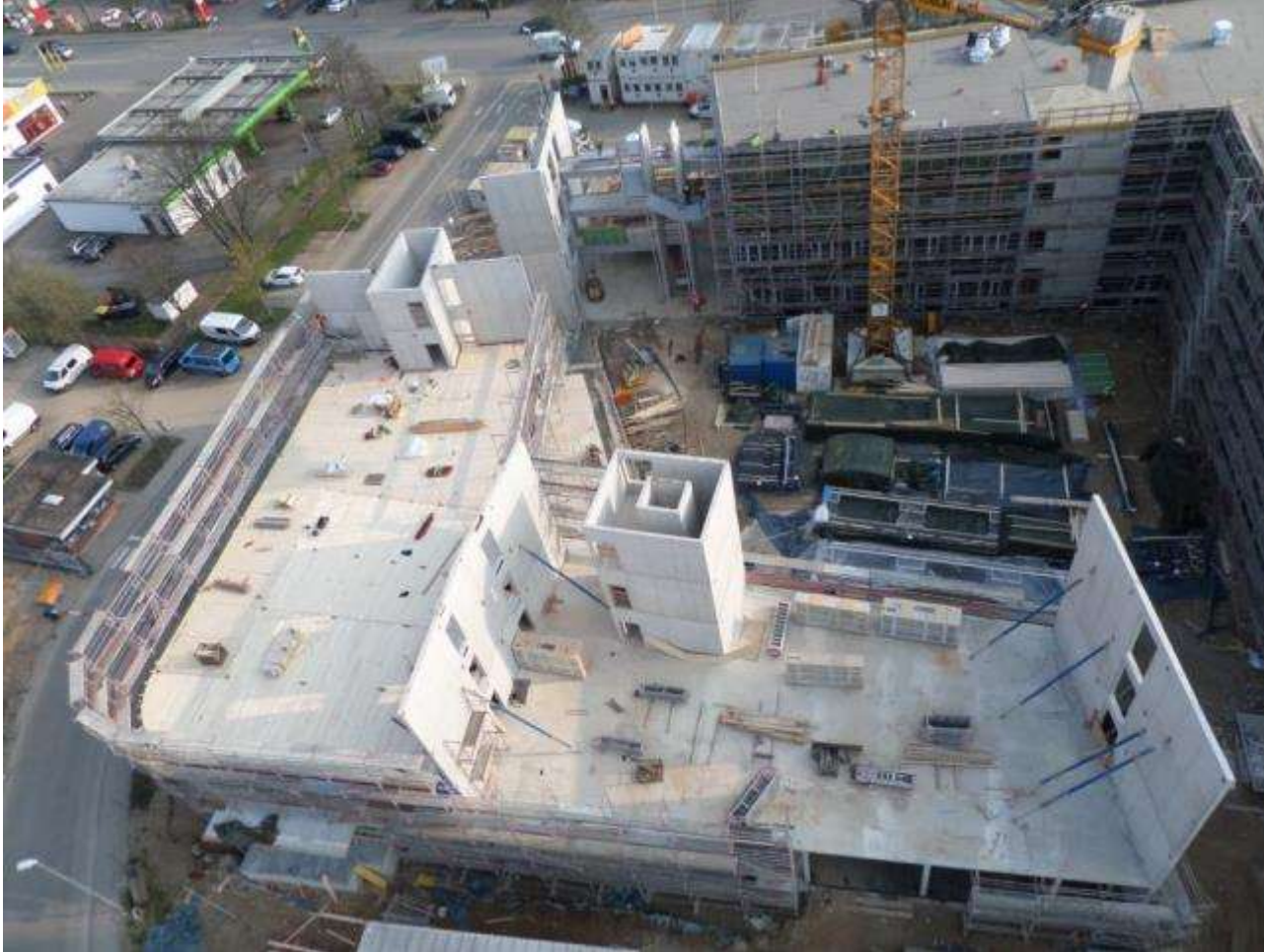
Site Situation 2 month after start
