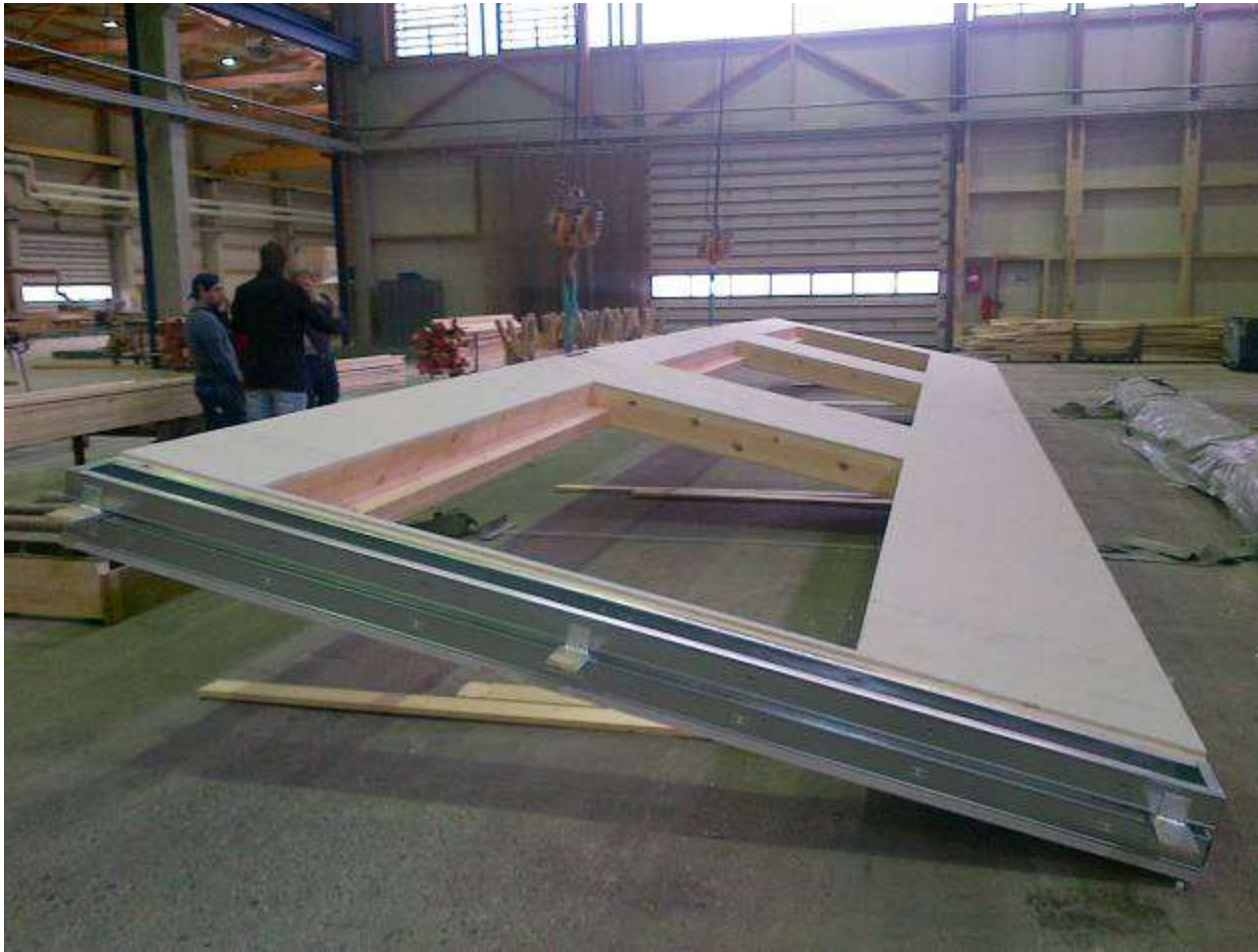
Prefabricated Wall panel 15 m long 3,60 high
