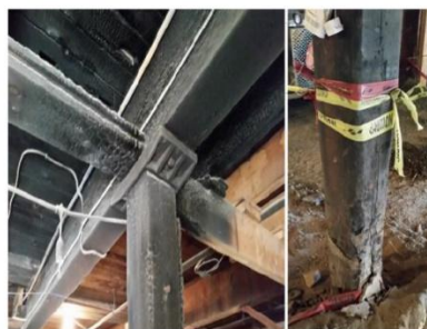
Figure 1. Fire-Damaged Column
