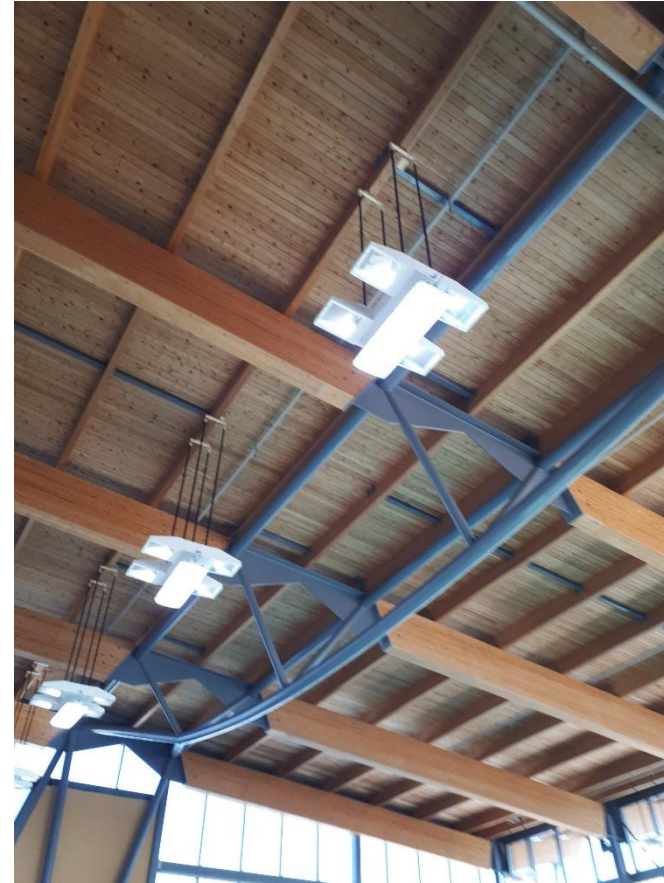
Steel truss and timber roof
