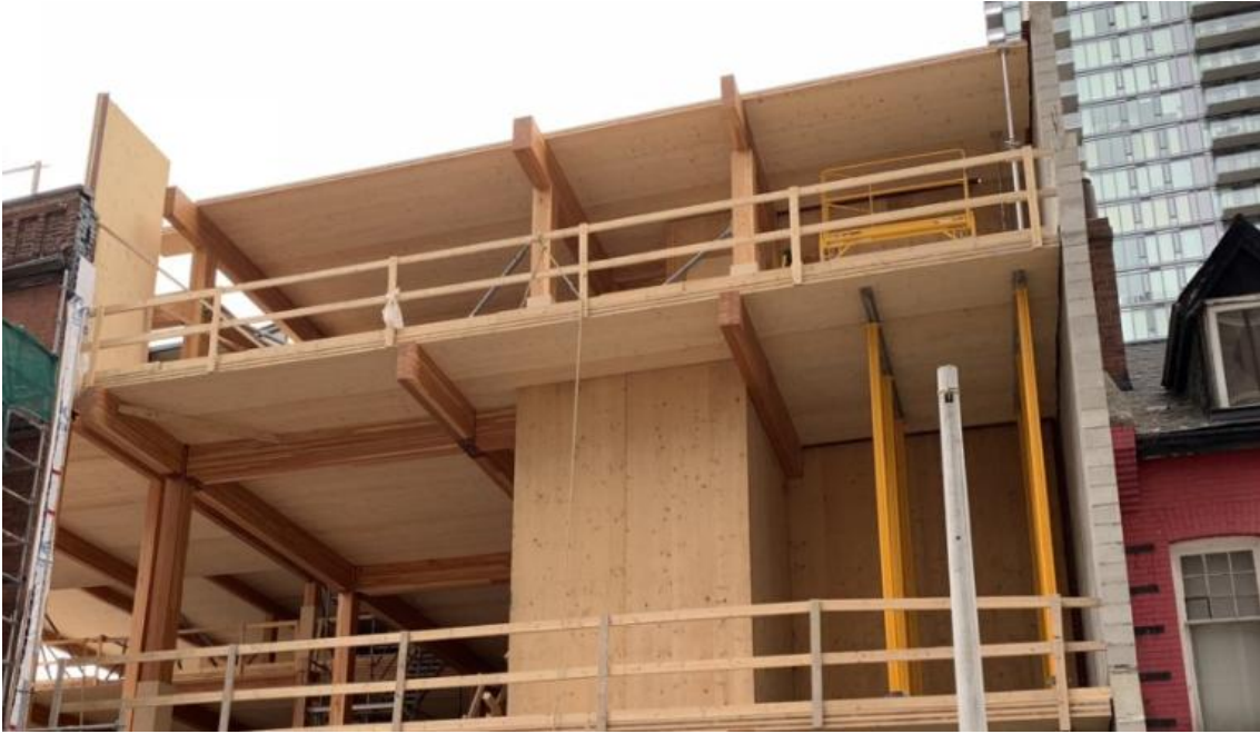
CLT paneling combined with glulam
