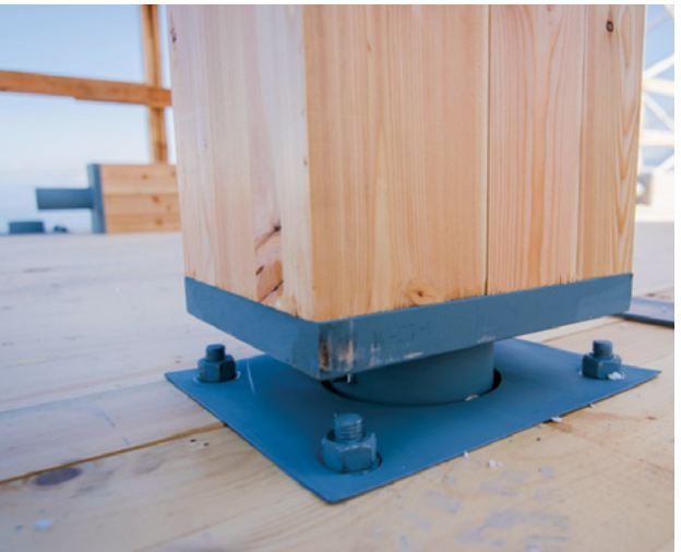
Custom steel connectors precision fit on-site
