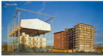
Temporary protective roofing at the Linnéplanen Hage construction site, Sweden.
