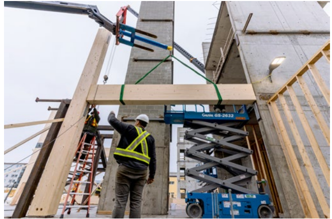
Figure 2. Beam installation between column and a concrete wall Photo Credit Jason Harding, courtesy of naturallywood.com
