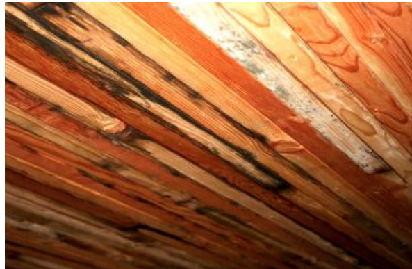
Figure 15. Moisture trapped in nail-laminated timber deck and causing damage (courtesy of SMT Research)
