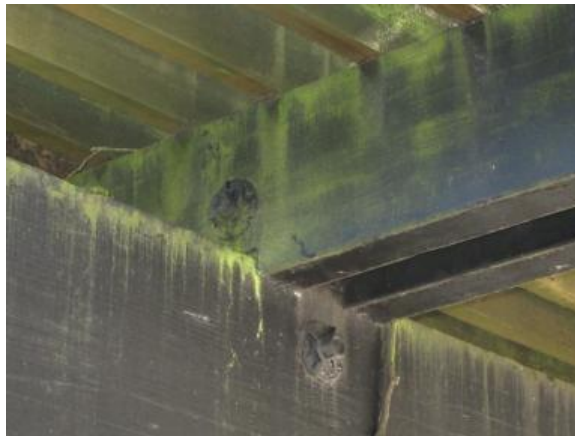
Figure 16. Crossing beams trapping water by capillarity showing up as algal stain
