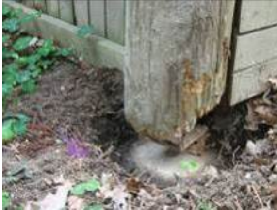
Figure 13. Rot in column base where soil level has risen.
