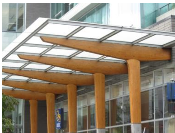
Figure 5. Exterior glulam on modern steel and concrete building protected by glass canopy, after 5 years without refinishing – well protected.
