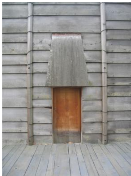
Figure 21. Weathered patina on naturally durable wood
