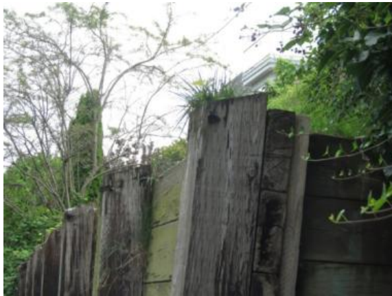
Figure 10. Rot (growing grass) in top of creosoted timber column cut at an angle
