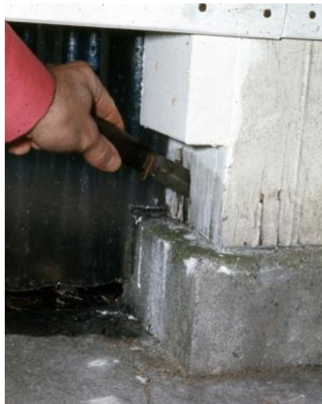
Figure 14. Rot in column base in direct contact with concrete.
