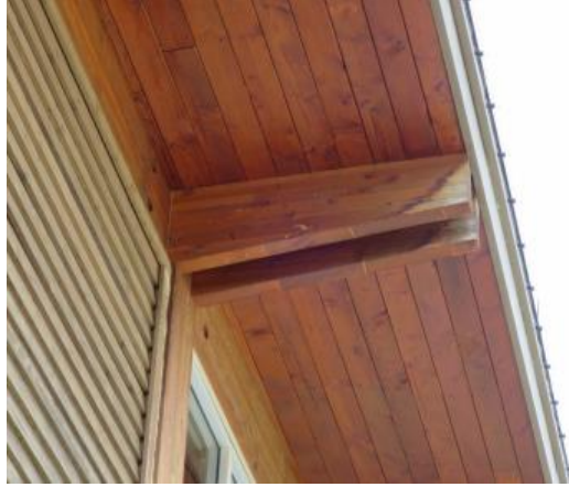
Figure 6. Inadequate overhang to protect beam from wind-driven rain leading to staining and coating failure on glulam ends
