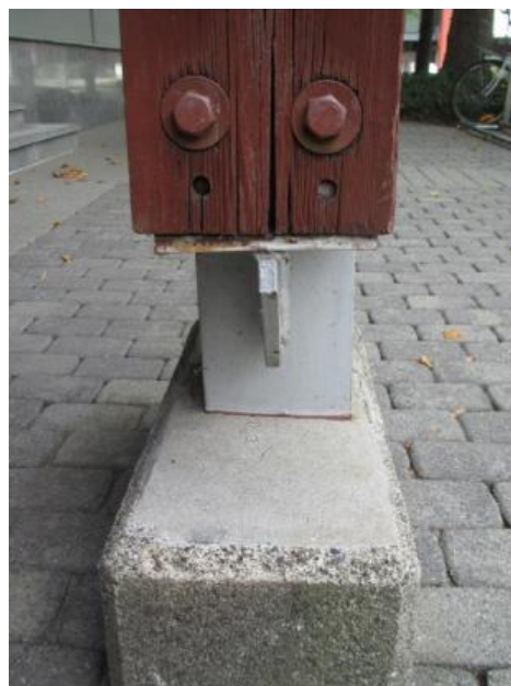
Figure 22. Borate rod placement between end grain and bolt holes
