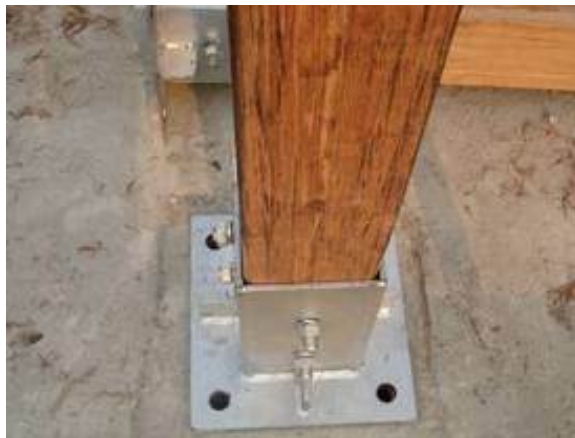
Figure 17. Metal boot around the base of a column is like putting wood in a bucket of water
