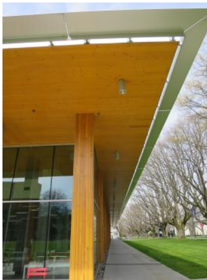
Figure 4. Exterior glulam and soffit on modern post and beam building under overhang – well protected.
