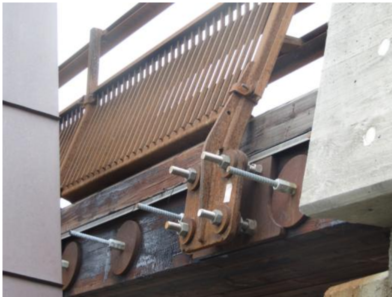
Figure 7. Metal plate connectors not too large to prevent drying on Sletta Bridge in Norway.
