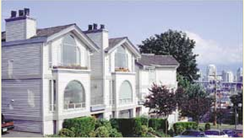
PHOTO 4: The Windgate townhouses near Choklit park in Vancouver, BC use decorative exterior fascia boards at the floor level, combined with sloping roofs and overhangs as part of a moisture management strategy.
