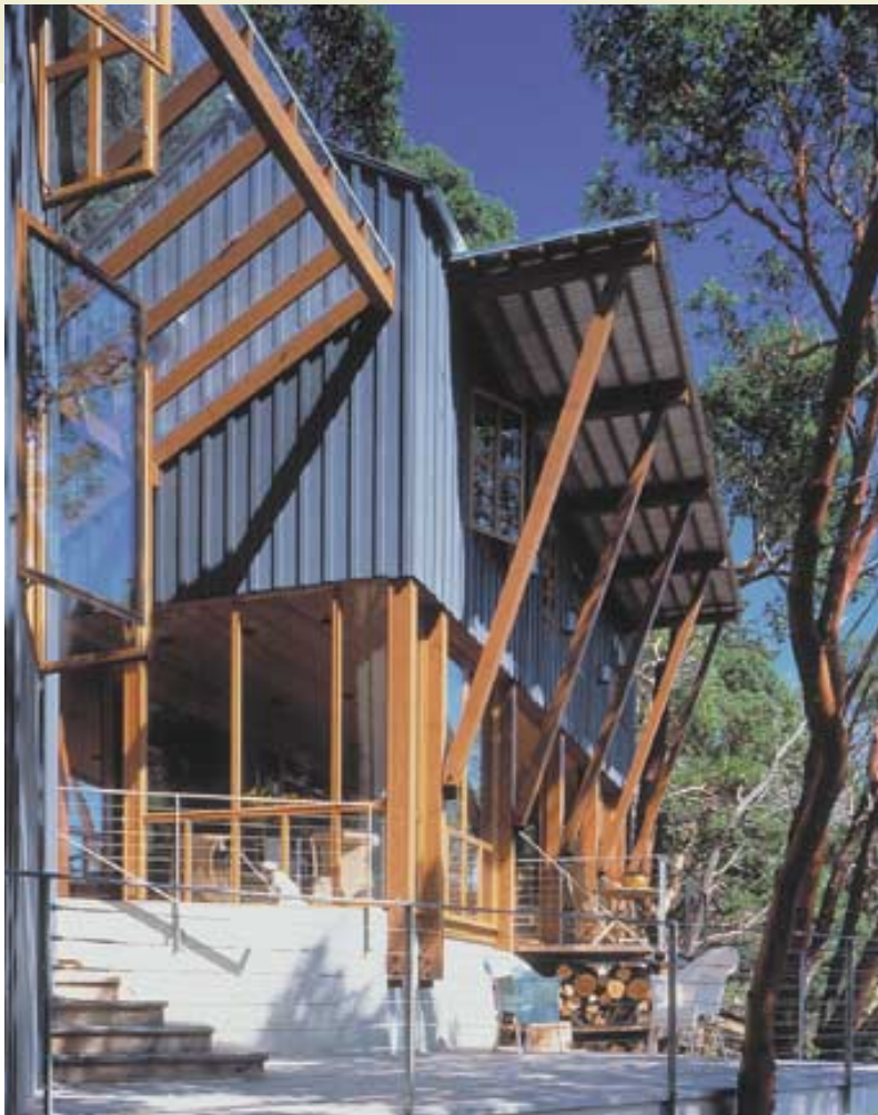
PHOTO 3: Girvin Cabin – This wood-frame studio and house located on Decatur Island, Washington uses pronounced overhangs that are both functional by deflecting rainwater from a window wall and architectural to suit the surrounding environment.
