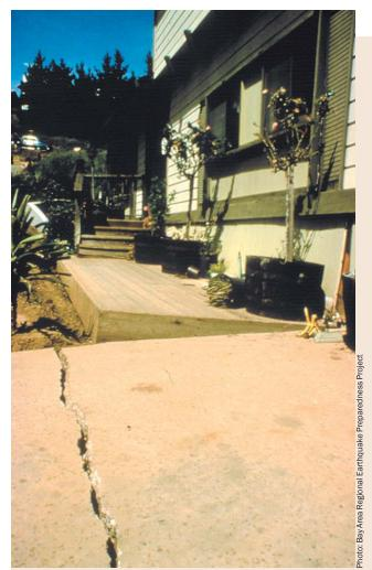
Exterior view of a wood-frame house illustrating damage caused by ground failure. Note cracks in the pavement at the front of the house.
