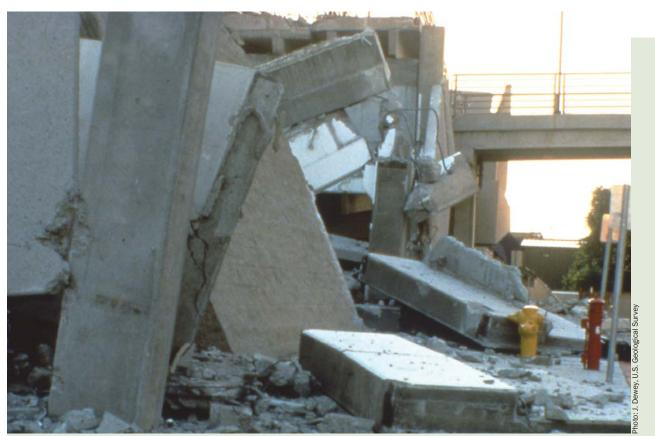
The second level of the concrete parking structure of the Northridge Fashion Center collapsed onto the lower level.
