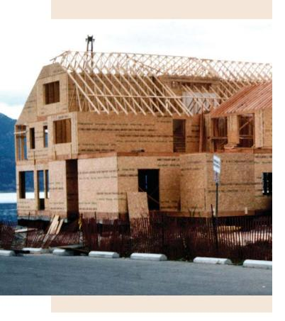
Wood-frame buildings have properties that naturally enhance their performance in earthquakes, although to ensure that wood-frame buildings are safe in earthquakes, good construction practices must be followed. Some of these properties are described in the following:
