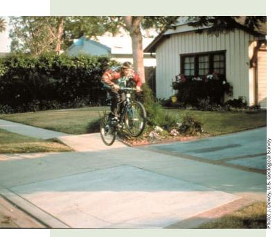
Overall wood-frame housing performed well in the Northridge earthquake. In front of this San Fernando Valley house, the sidewalk tented due to strong ground shaking although the house did not sustain visible damage.
