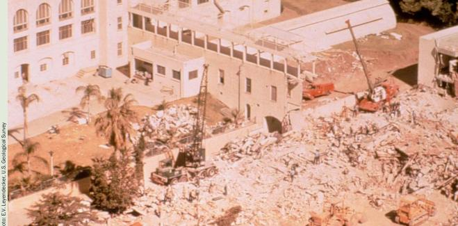
Aerial view of the damage to the San Fernando Veterans Administration Hospital and complex. The collapsed masonry structure was built in 1926, before earthquake building codes were in effect. Forty-seven deaths occurred as a result of the collapse of the structure.
