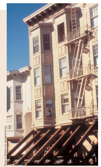
Shored building in the Marina District of San Francisco following the 1989 earthquake. Note the garage area on the first floor beneath the apartments that created a weak first storey.
