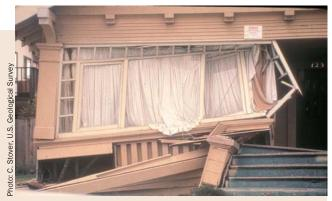
Failure of cripple wall in the Loma Prieta Earthquake.
